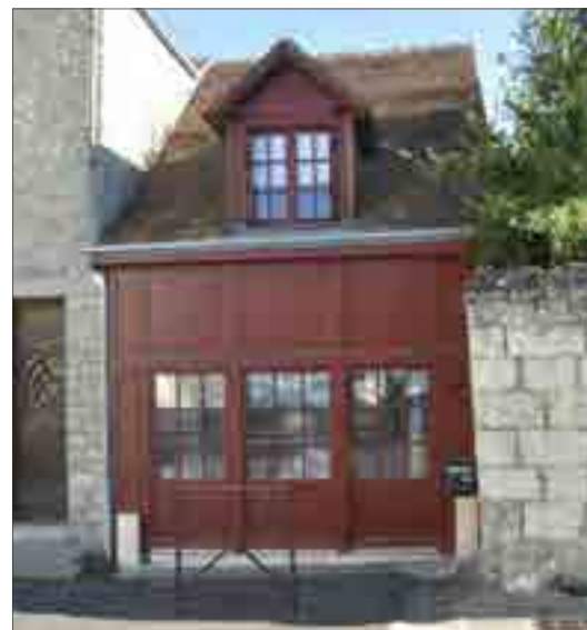
Fig.225 : Façade place Mazerolles
